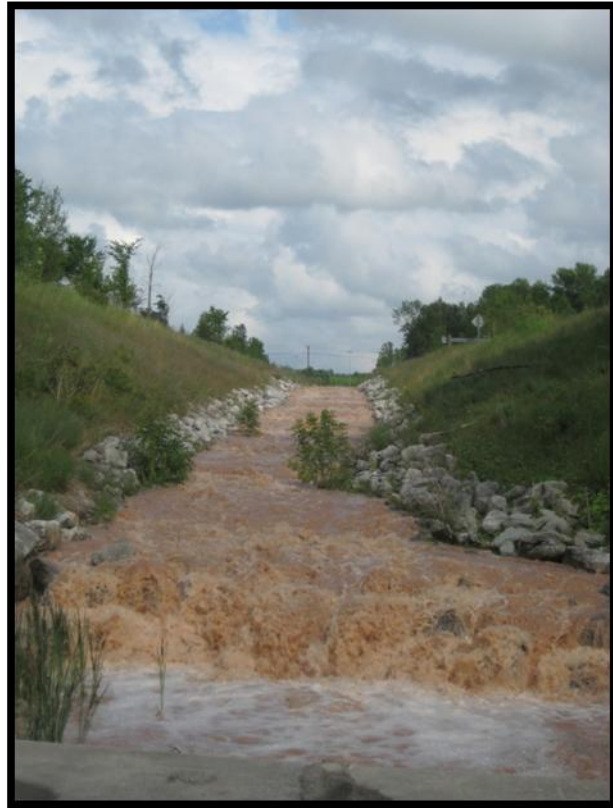
Figure 3: Under high flows, municipal drains and storm sewers can rapidly move contaminants toward a surface water intake. (SGSNBP Source Protection Region)
