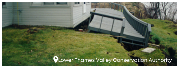
Slope Failure
