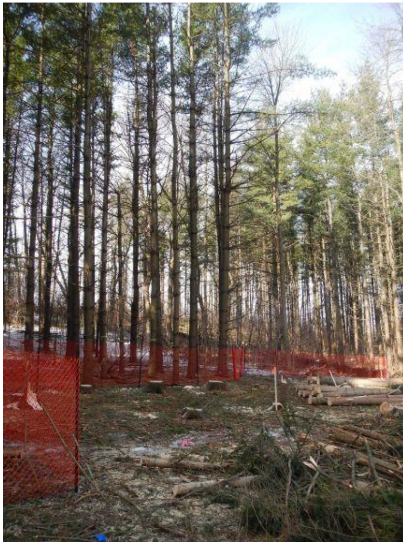
Cultural plantation clearing and protection (Credit: City of Guelph)
