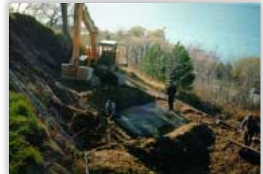
Figure 85 - Installation of Geomattting
