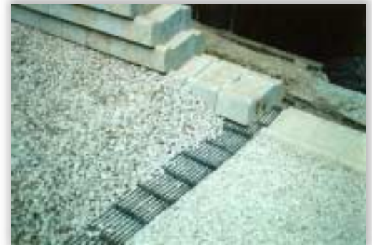
Figure 86 - Drainage Designed by Geotechnical Engineer
