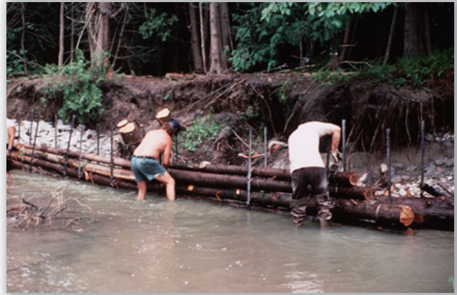
Figure 133 -Installation of Log Crib
