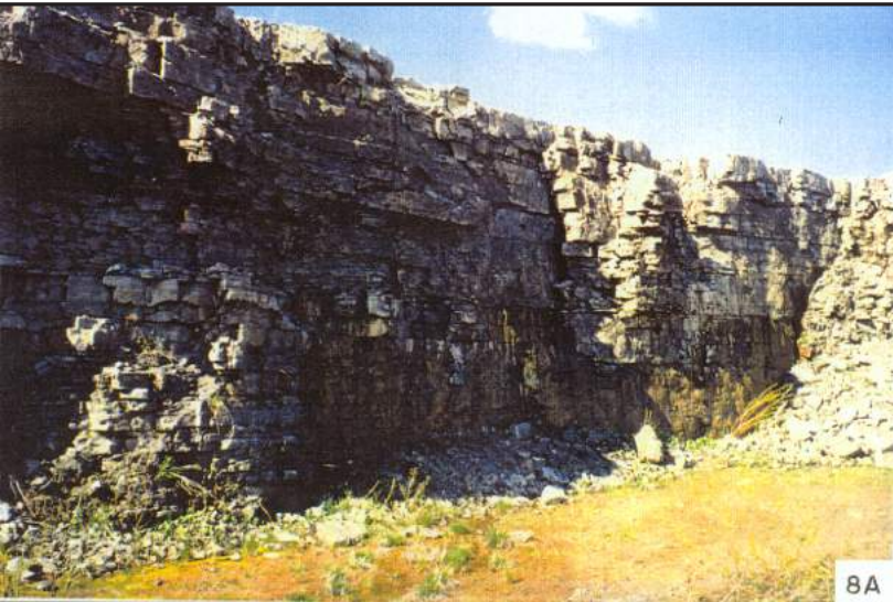
Figure 5.5: Bedding Seepage - Flamboro Quarry (Plate 8)
