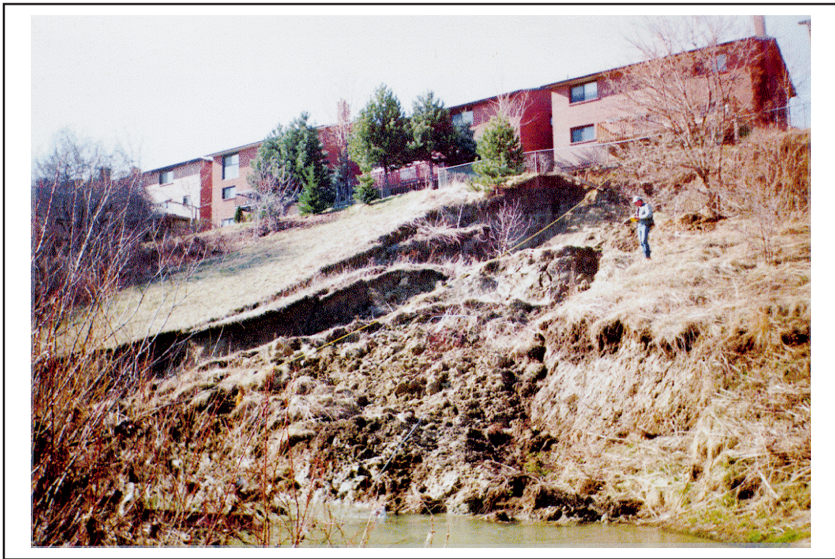
Figure 4.9: River Bank Erosion
