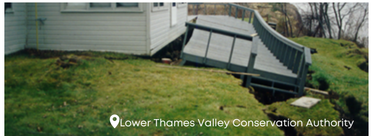
Slope Failure
